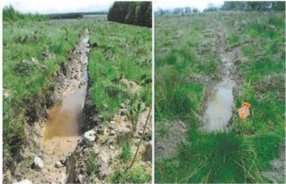
In-drain sediment trap (left) and a sediment trap adjoining a water setback (foreground) (right).
